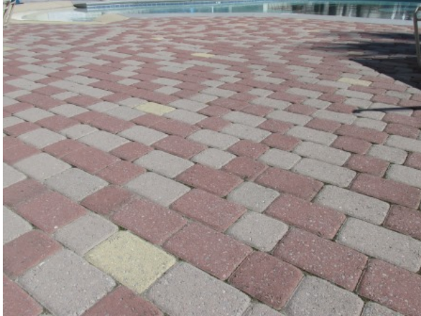
Masonry deck pavers
