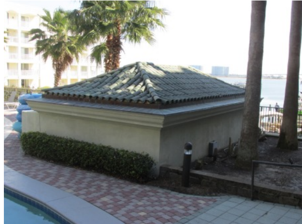
Pool storage concrete tile roof
