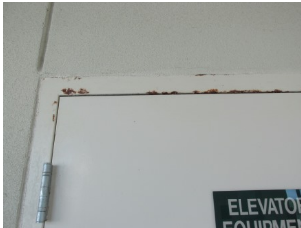
Isolated rust at common door
