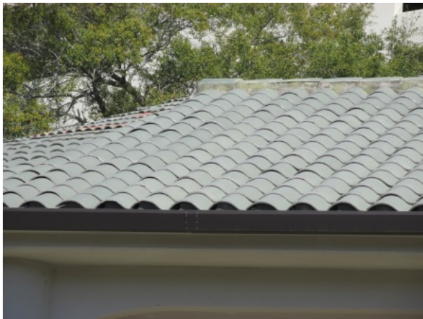
Porte cochere concrete tile roof
