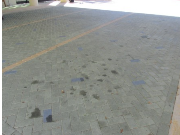
Masonry pavers at the porte cochere
