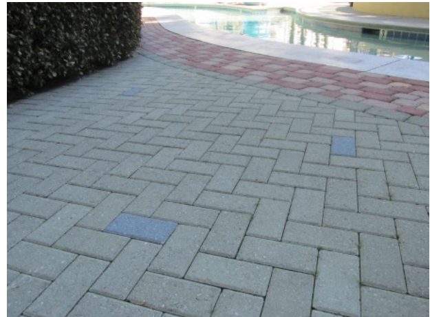
Masonry deck pavers
