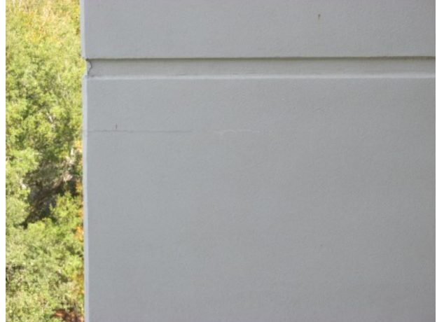
Stucco crack
