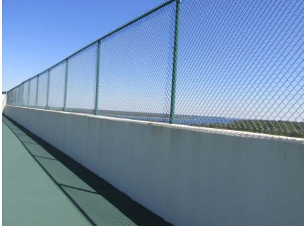
Tennis court fence
