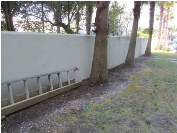
Perimeter wall overview
