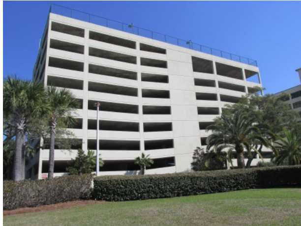
Parking garage overview
