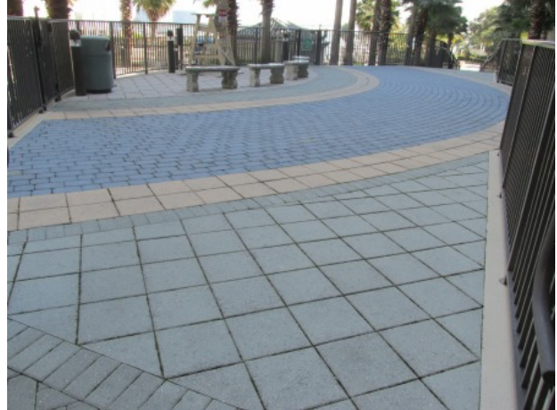
Masonry deck pavers
