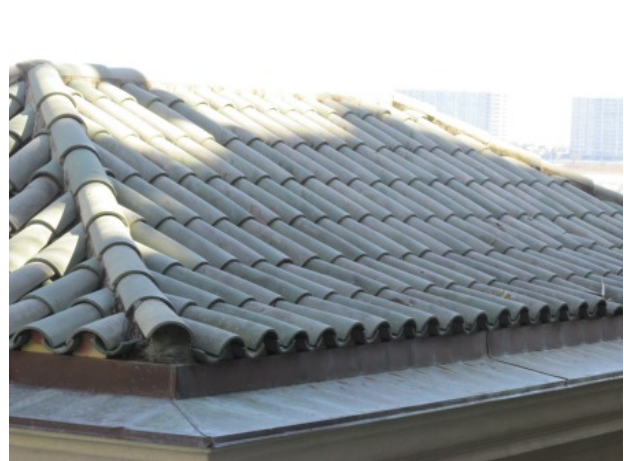
Pool storage concrete tile roof
