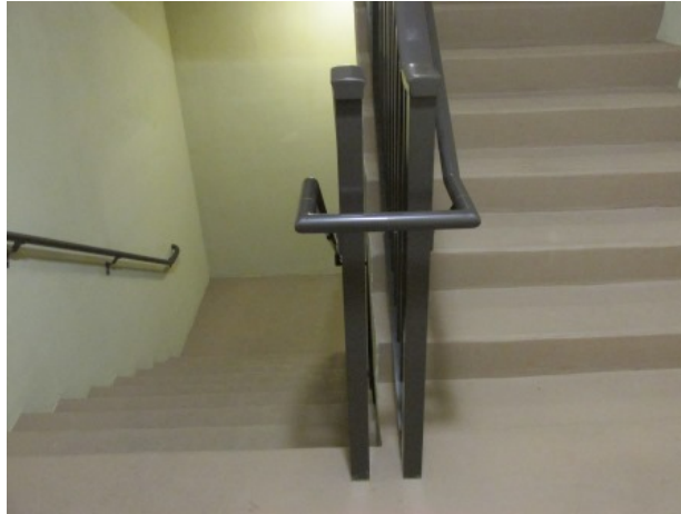
Stairwell paint finishes
