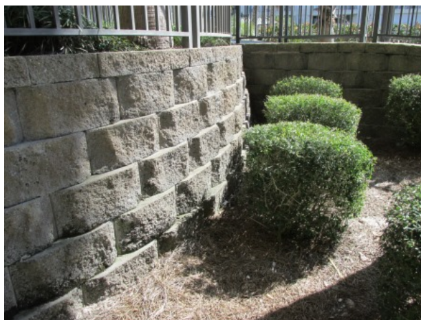
Masonry retaining wall
