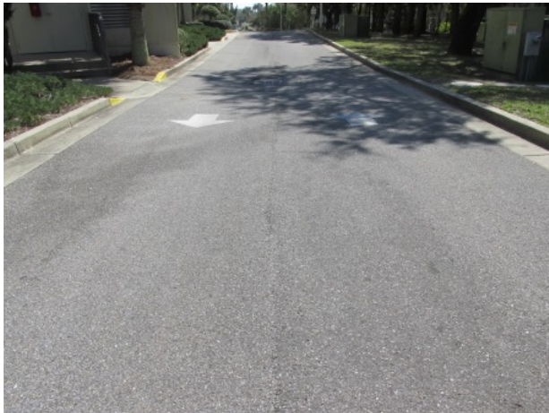
Asphalt pavement overview
