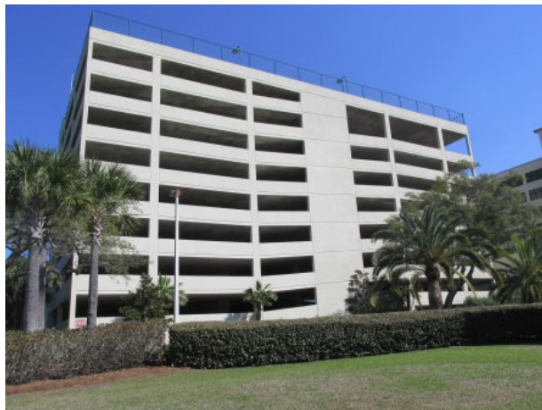
Parking garage overview
