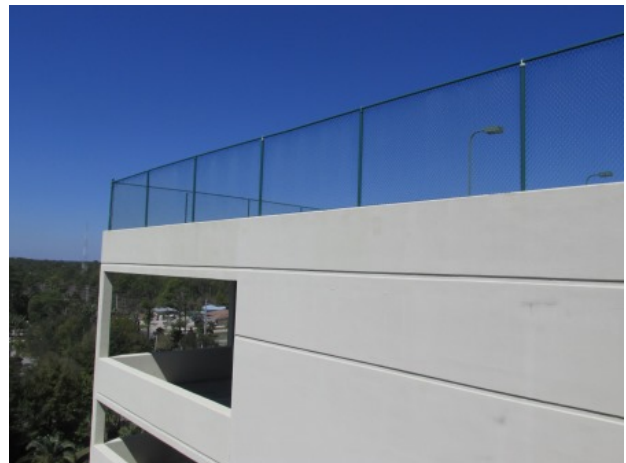
Parking garage stucco paint finish
