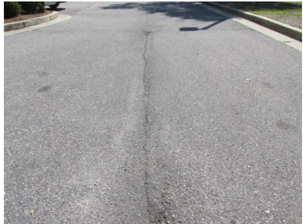
Centerline crack
