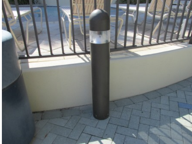
Typical bollard light fixture
