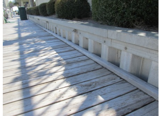
Old steel bulkhead
