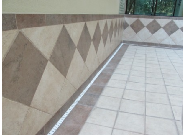
Wall tile at indoor pool
