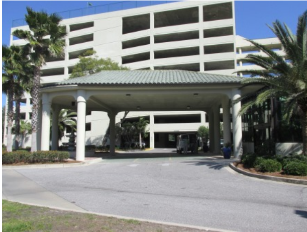
Porte cochere concrete tile roof
