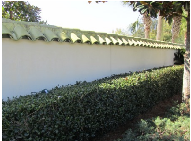
Perimeter wall near entrance
