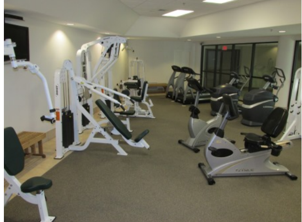
Exercise room carpet – note stains
