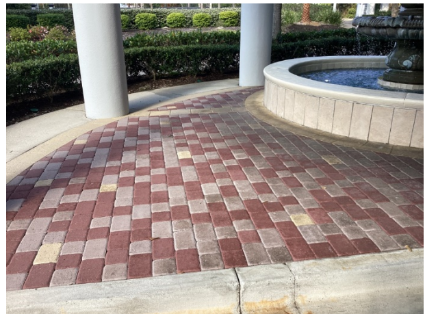
Masonry pavers overview
