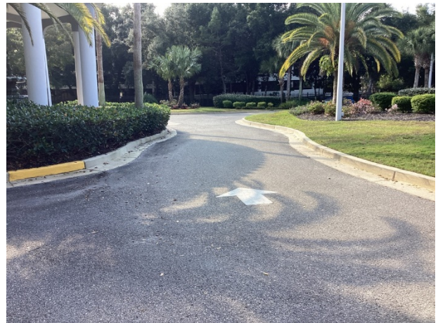
Asphalt pavement street overview
