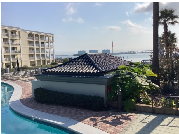
Concrete tile roof
