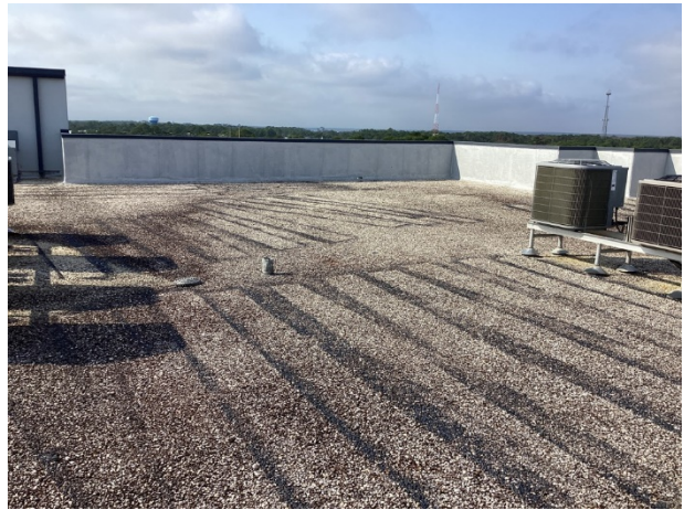
Built-up roof overview
