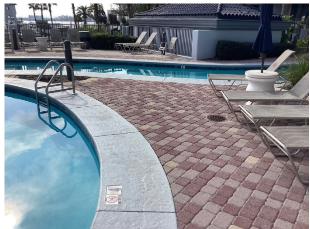
Paver pool deck overview
