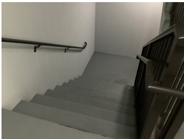
Stairwell paint finishes
