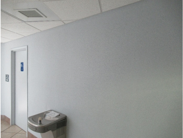
Overview of interior paint finishes
