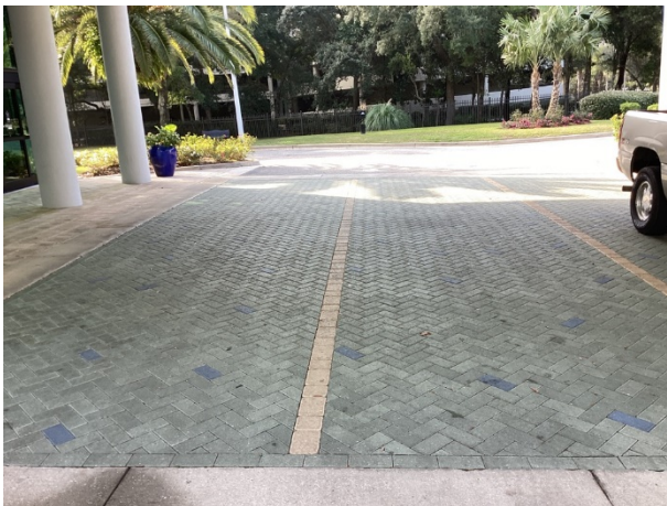
Masonry pavers overview
