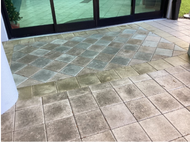
Masonry pavers overview
