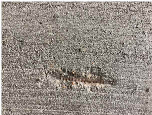
Exposed reinforcement
