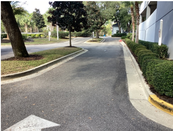
Asphalt pavement street overview
