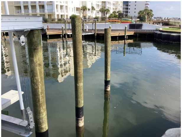
Overview of wood pilings
