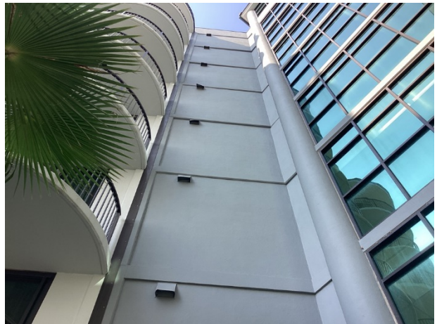
Stucco wall finishes
