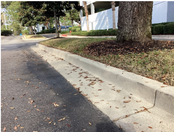
Concrete curb and gutter
