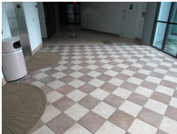
Overview of tile floor coverings
