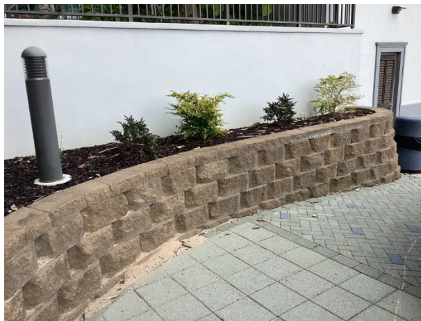
Masonry retaining walls overview
