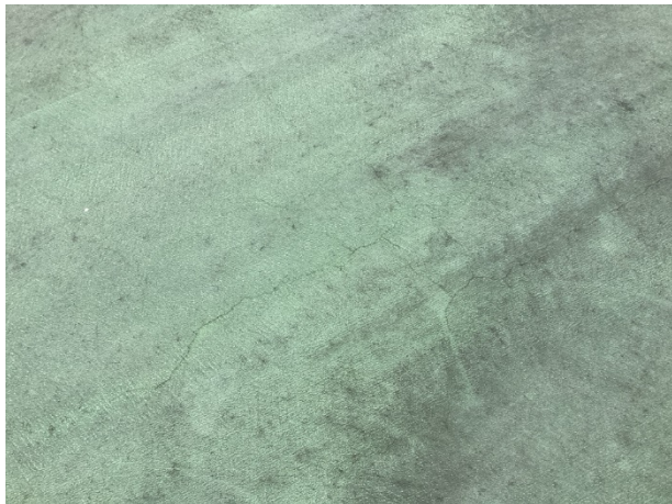
Surface cracks
