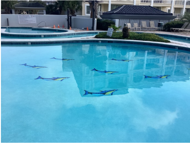
Pool plaster overview
