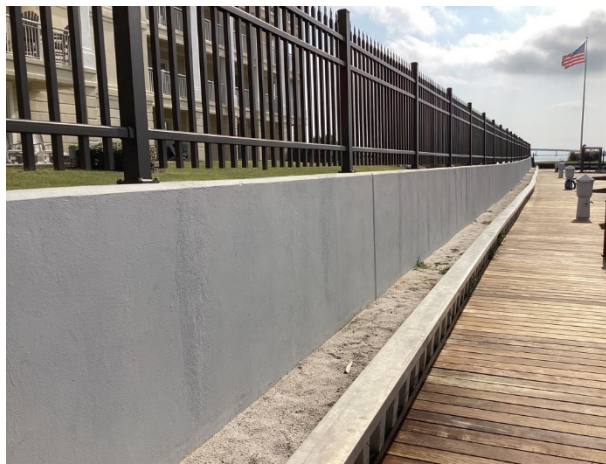
Concrete retaining walls overview
