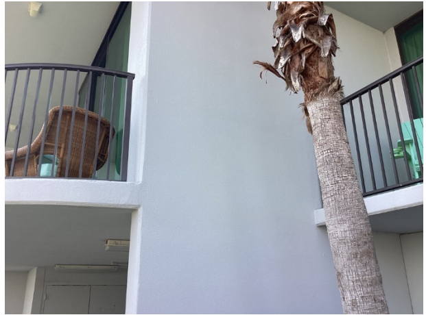
Stucco wall finishes
