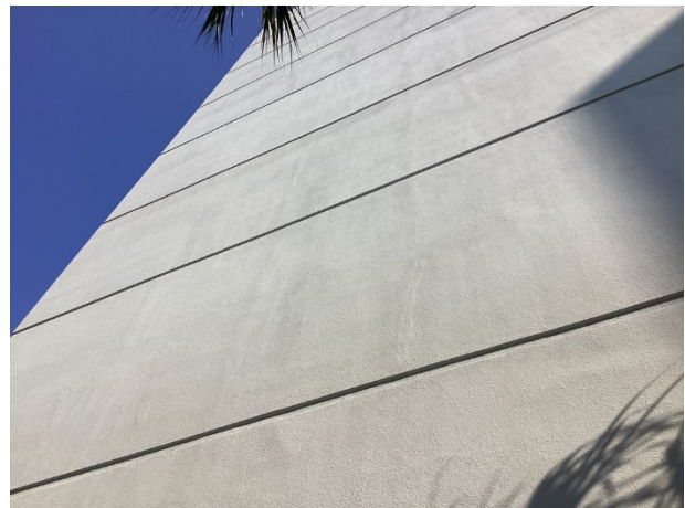
Stucco wall finishes
