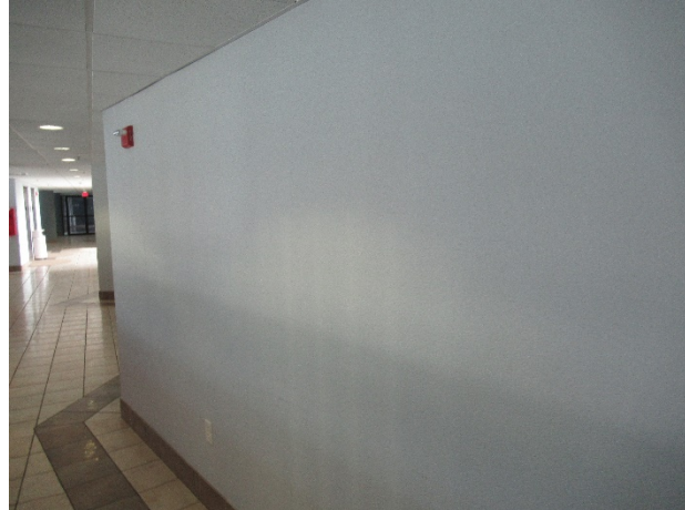
Overview of interior paint finishes
