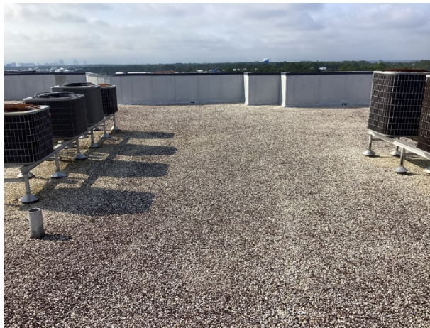
Built-up roof overview
