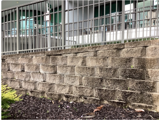
Masonry retaining wall
