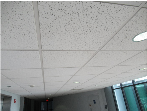
Overview of acoustic ceiling tiles
