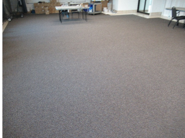
Overview of carpet floor coverings
