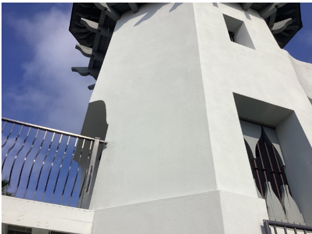
Stucco wall finishes
