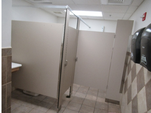
Overview of restroom
