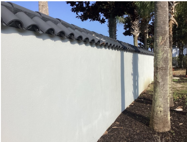
Stucco perimeter wall overview
