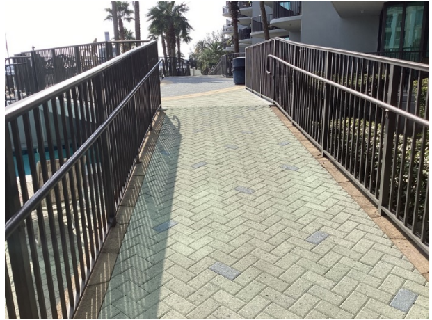
Paver pool deck overview
