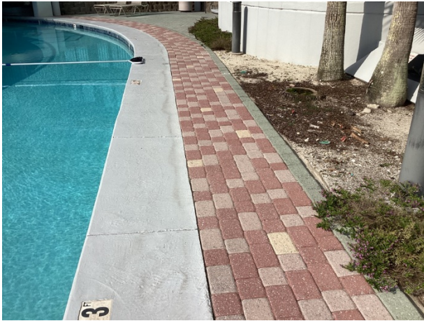
Paver pool deck overview
