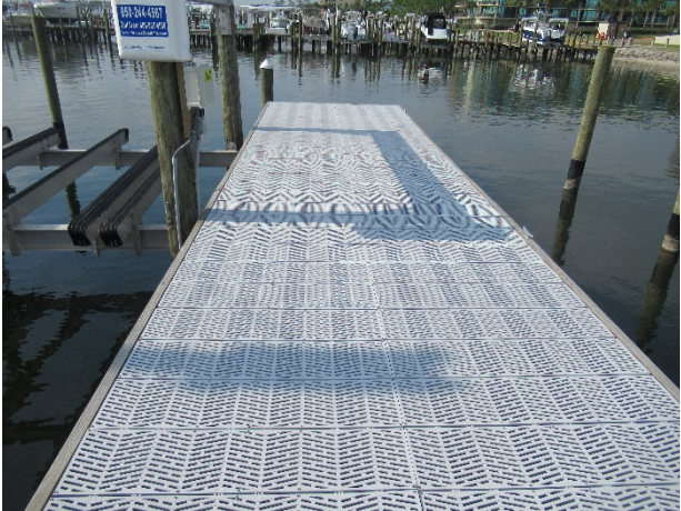
Dock with composite decking
