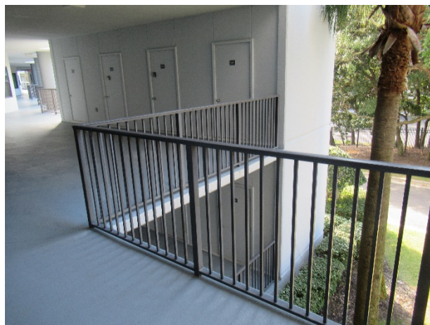
Overview of railings
