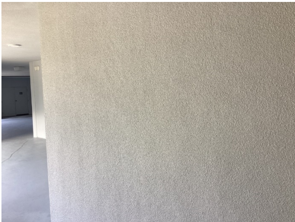
Stucco wall finishes
