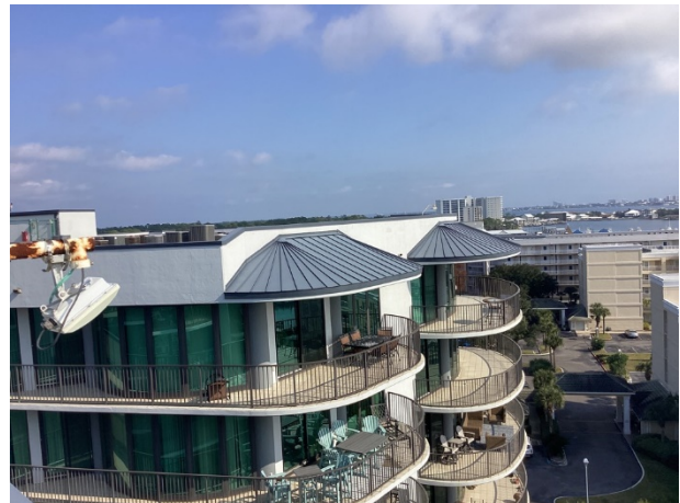
Metal roofs overview
