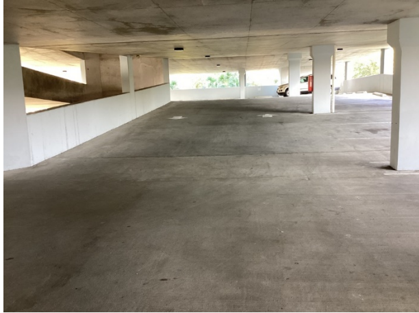
Elevated garage floor overview
