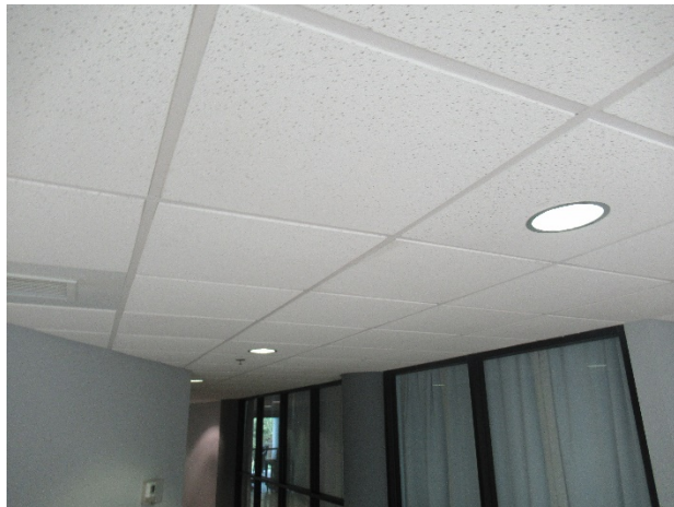
Overview of acoustic ceiling tiles
