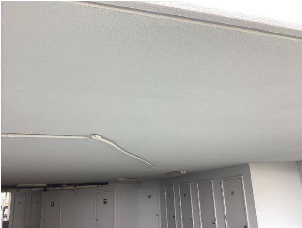
Stucco wall finishes
