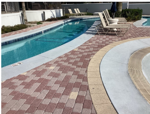
Paver pool deck overview
