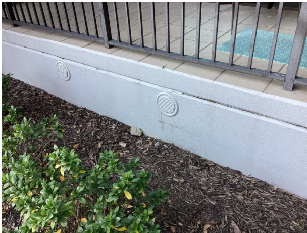
Stucco cracks
