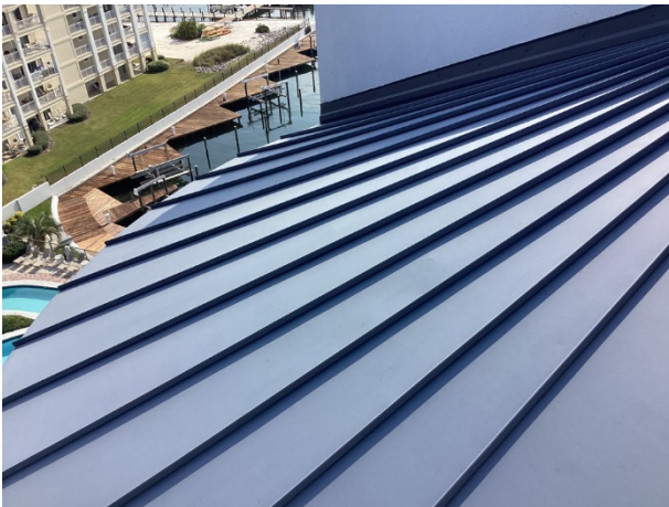
Metal roofs overview
