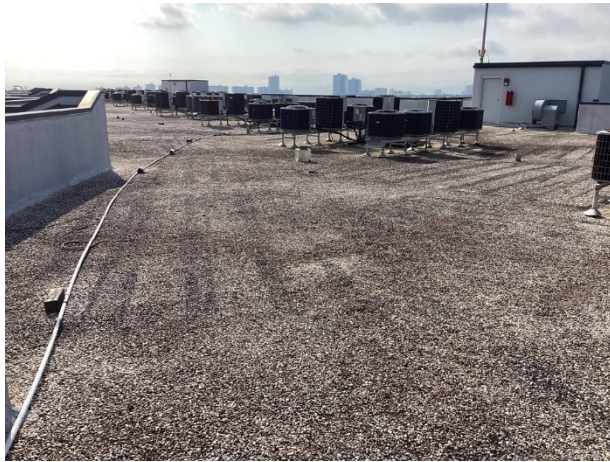
Built-up roof overview
