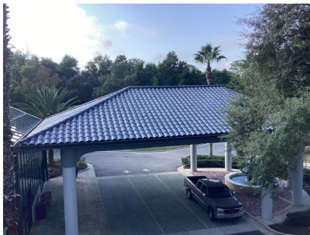
Concrete tile roofs overview
