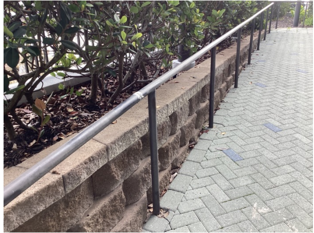
Masonry retaining walls overview
