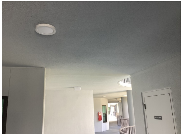
Stucco wall finishes
