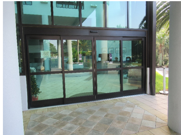
Lobby area entrance doors
