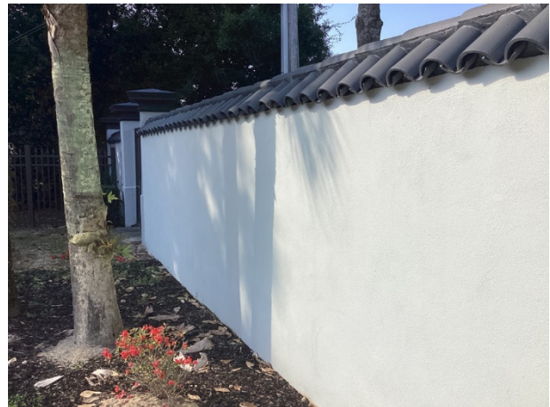
Stucco perimeter wall overview
