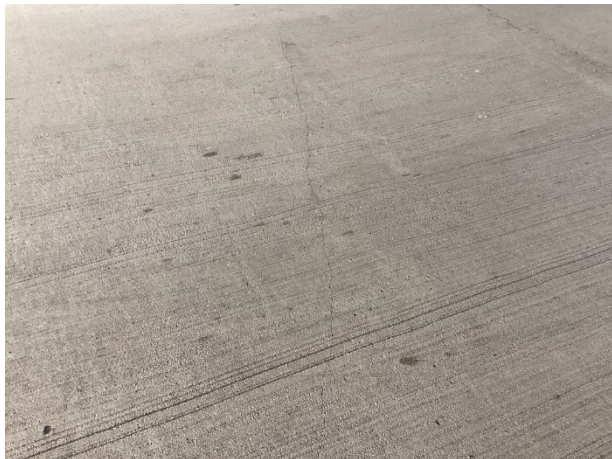
Concrete cracks
