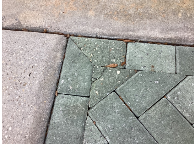
Paver cracks
