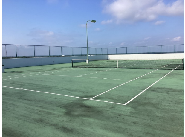
Tennis court overview
