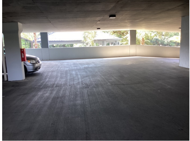
Elevated garage floor overview
