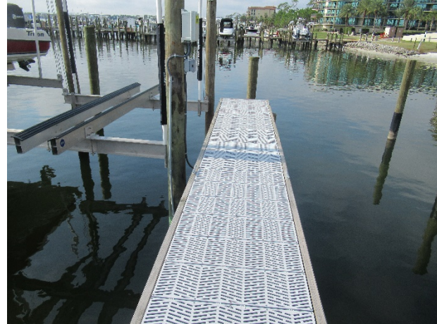
Dock with composite decking
